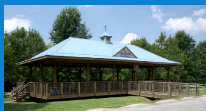
Pearsons Springs Pavilion
